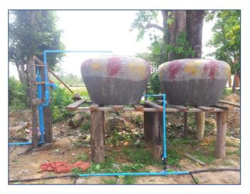
Connection of water-pipe system, pcv pipe, pump and water jars
